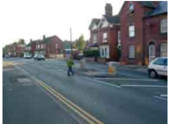
Figure 6/1 – Pedestrian Refuge Island on A49 in Hereford
