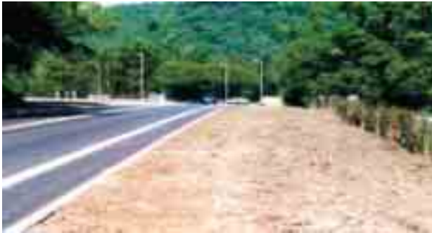
Above: Typical verge situation showing wide area which could comfortably accommodate a new pedestrian and cycling route. It is also sufficient to accommodate pedestrians & horses in an OCR.
