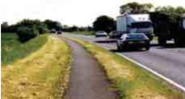
Above: An existing path of 1.0m is already separate from the road, but at a distance less than the recommended 1.8m for equestrian use (see TA 90). The verge on the left would comfortably accommodate a wider path and allow the existing grass verge to be widened to 1.8m.
